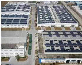
Hubei Huangshi Rifeng Project China System Capacity: 3.1 MW
