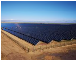
Agadyr Power Plant Kazakhstan System Capacity: 50 MW
