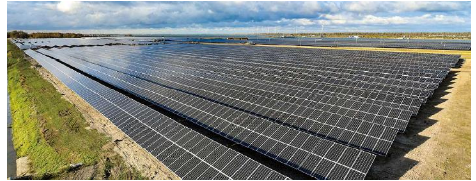
Shell Moerdijk Power Plant Netherlands System Capacity: 26.6 MW
