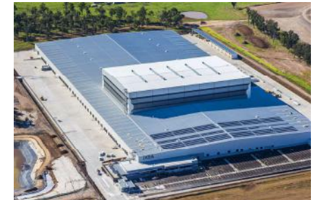
IKEA Rooftop Project Australia System Capacity: 384 KW
