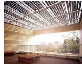
Kowa Elementary School BIPV Project Japan System Capacity: 10 KW
