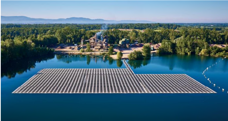
Baggersee Maiwald Floating Power Plant Germany System Capacity: 750 KW
