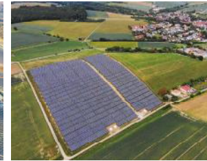
Bejulo Solar Power Plant Germany System Capacity: 58.3 MW
